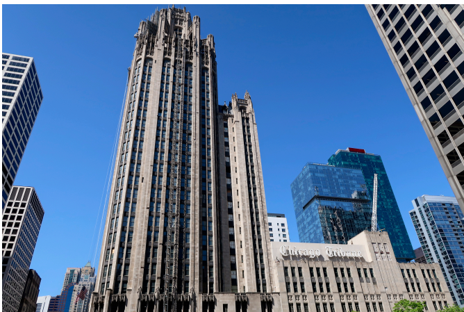
Work begins in 2019 on the Tribune Tower's luxury condo conversion. The renovated landmark boasts new shops, restaurants, and a Museum of Ice Cream. Photo: Bex Walton/Creative Commons.
