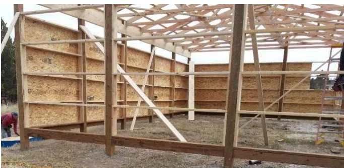
Blue Sky Building Supply pole building under construction
