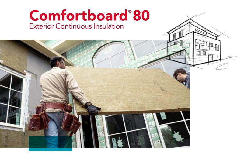
ROCKWOOL Comfortboard® 80 thermal insulated sheathing is a rigid stone wool insulation board designed for use as an exterior continuous insulation. Comfortboard® 80 does not produce smoke or propagate flames, keeping occupants safe and reducing property damage in the event of a fire. Vapor permeable, this solution allows fast outward drying, keeping moisture out of your wall assembly.
