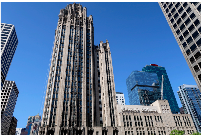
Work begins in 2019 on the Tribune Tower's luxury condo conversion. The renovated landmark boasts new shops, restaurants, and a Museum of Ice Cream. Photo: Bex Walton/Creative Commons.
