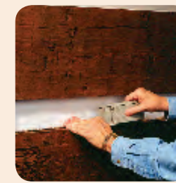
2. Tape the entire joint using polyester tape.
