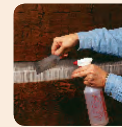
4. Lightly mist the trowel as needed.
